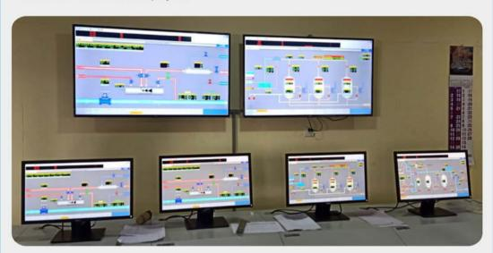
Bestway formerly known as (MCL) DCS revamping project is the biggest project of CSE in Pakistan till now. We offered the latest developed WebField ECS-100 DCS consisting of 7 Control Stations, 9 Operator Stations, 2 Engineer Station, and 2 redundant Data Servers. The total I/O quantity reaches to 6,954, and other 3,776 points were integrated in the system through Profibus DP communication interfaces.
